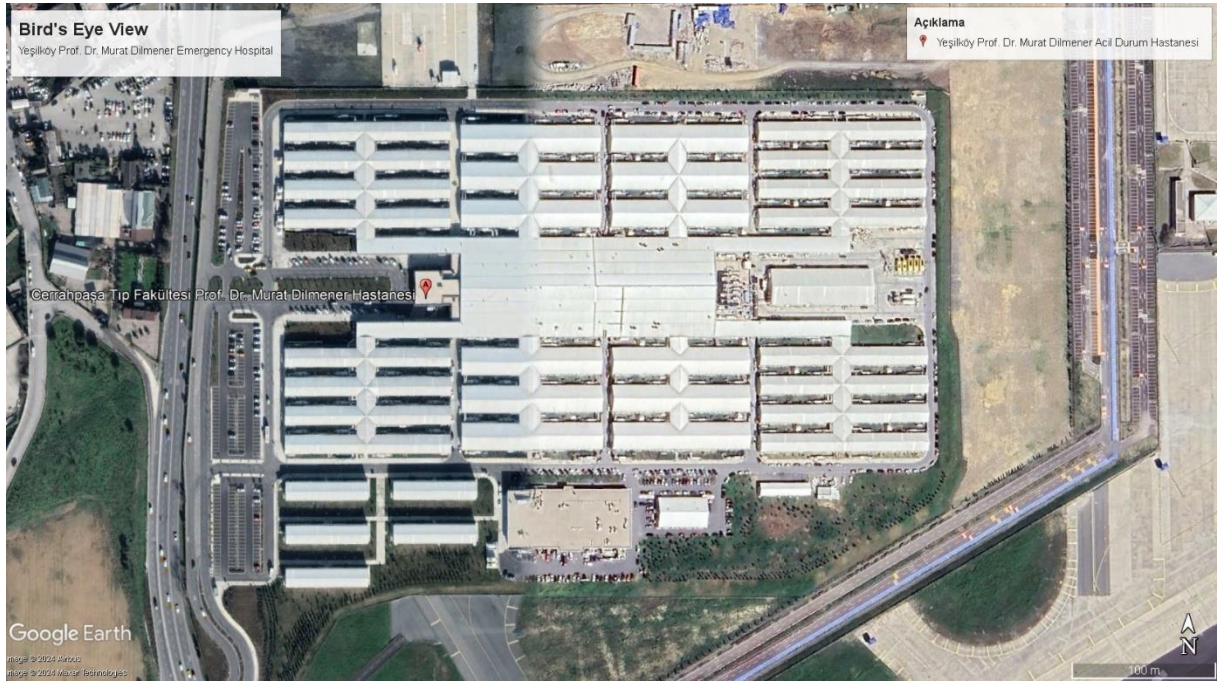
Figure 2. Satellite image of the case study hospital
